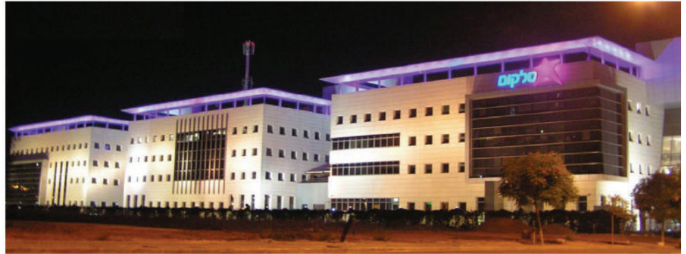
Cellcom Telecommunications, Inc. • Netanya, Israel
